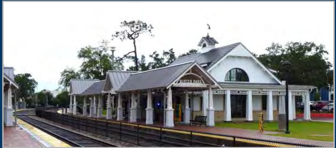
Winter Park, FL (2014): Platform with canopy, attached waiting area, restrooms ($1.2 million)
